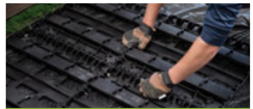
Step 1. Ensure a flat, level surface and set tiles
