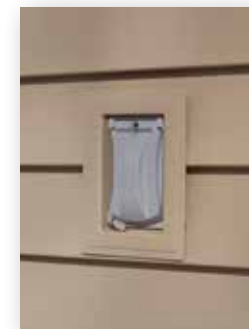
Recessed Electrical Blocks
