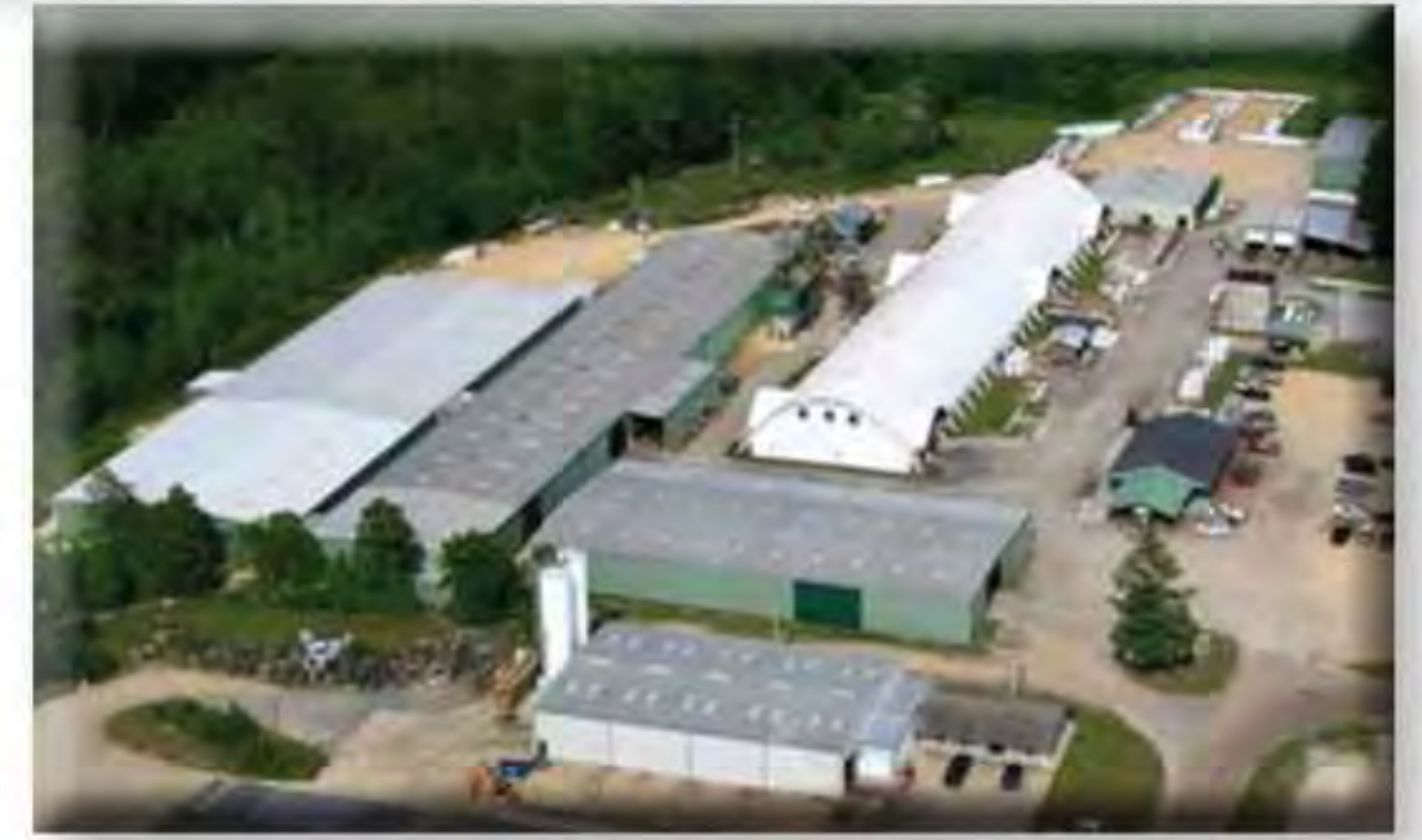
Laminating Plant - El Dorado, AR
