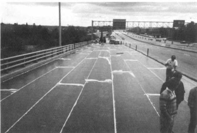
Approximately 500,000 sq. ft. of waterproofing membrane installed on the Piscataqua River N.H./Maine bridge.
