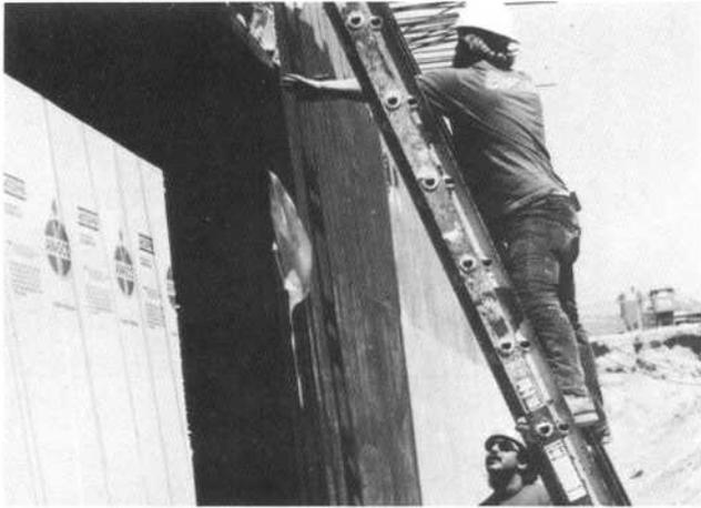
Carnation office building project. 46,200 square foot foundation waterproofing, Pasadena, California. Eberhard Roofing, approved installer. Note: Protection board can adhere to membrane without adhesives.
