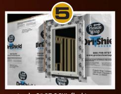
Apply 9" BT-25XL flashing over side jambs and head of window to complete installation.
