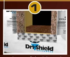
Apply BT25XL flush with the top edge of the sill, extend beyond rough opening equal to the width of the flashing.
