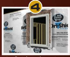
Install window with a continuous 3/8" bead of Protecto Sealant 25XL behind nailing flange.
