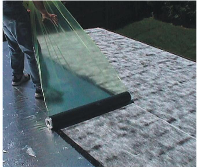
laps, position the sheet, even remove and reposition the membrane in case of error without struggling with the entire peel and stick adhesive backing.
