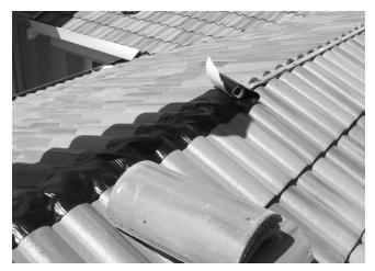
Center the material on the ridge of hip board and loosely lay the tape so there is a slight sagging down into the pans of the tile.
