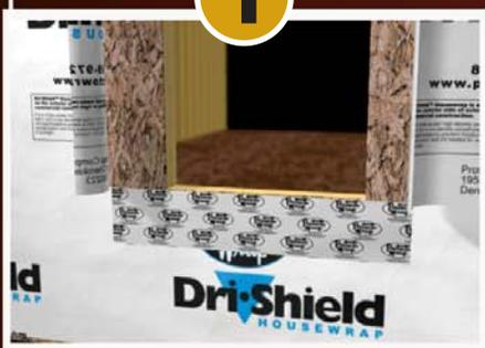
Apply BT25XL flush with the top edge of the sill, extend beyond rough opening equal to the width of the flashing.
