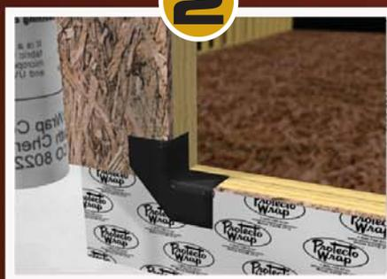
Remove release liner and apply the detail tape in each corner of the rough opening. Fold out over the BT25XL.
