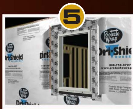
Apply 9" BT-25XL flashing over side jamba and head of window to complete installation.
